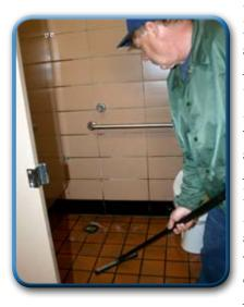
the low-flow/ low-pressure spray nozzle. After cleaning, the solution is rinsed away with water from the spray nozzle. Any remaining liquid can be maneuvered into a floor drain with a squeegee or mopped dry. An optional
